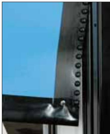
Spaced just 1.5 inches apart, the drive spheres provide tension along the entire curtain.
